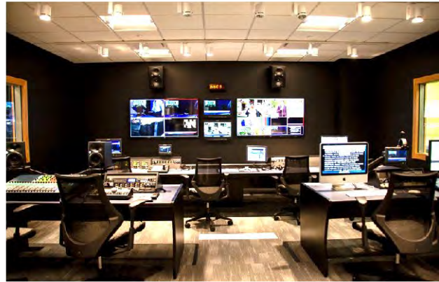
Video Control Room
